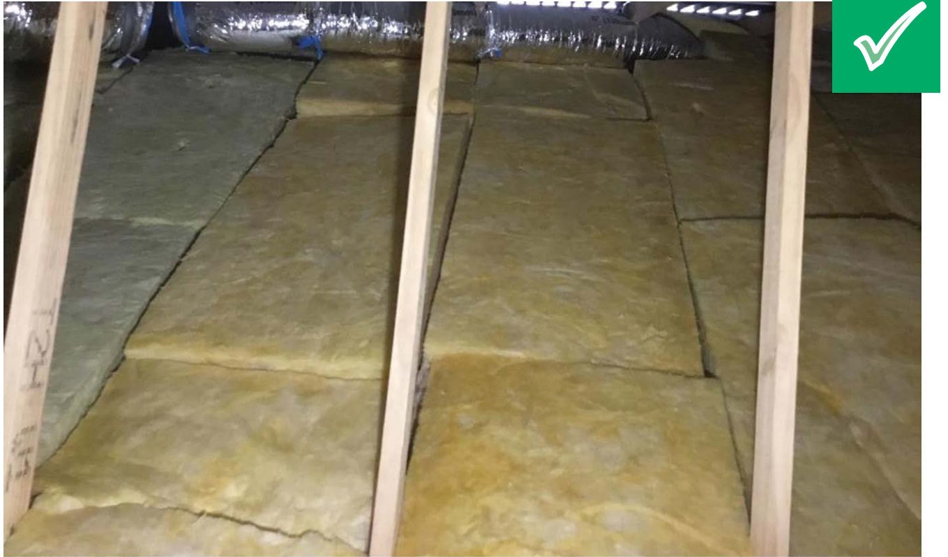
Figure 2. well-installed ceiling insulation
